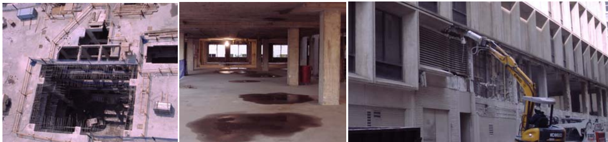
Figure 1: Illustration of demolition on WestEnd25
