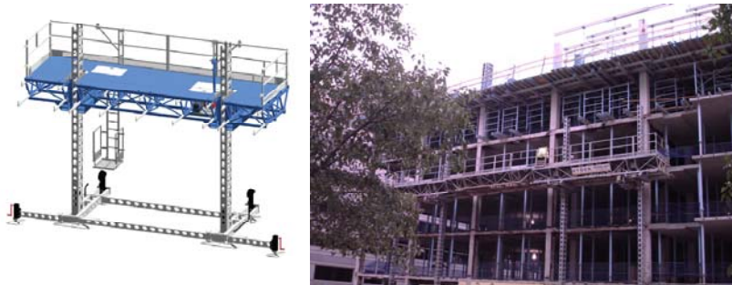
Figure 3: Hydraulic Mast Climbing Scaffold System for Masonry Installation
